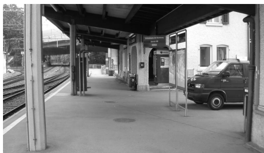
Figure 4.1 An unconscious link or ULINK connects two spaces without being consciously experienced when moving from one space to the other. In the image, the platform is connected to the small square (where the van stands) by means of a ULINK . Unconscious links have no physical manifestation.
